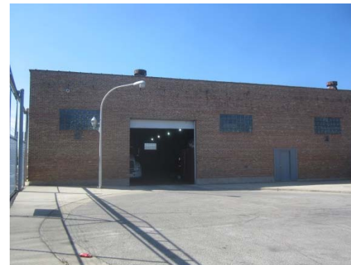
Existing warehouse entrance on Lockwood
