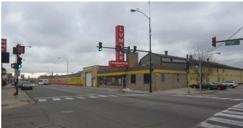
Existing lumberyard at Grand Ave and Long Ave
