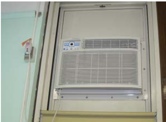
Typical Window A/C Installation
