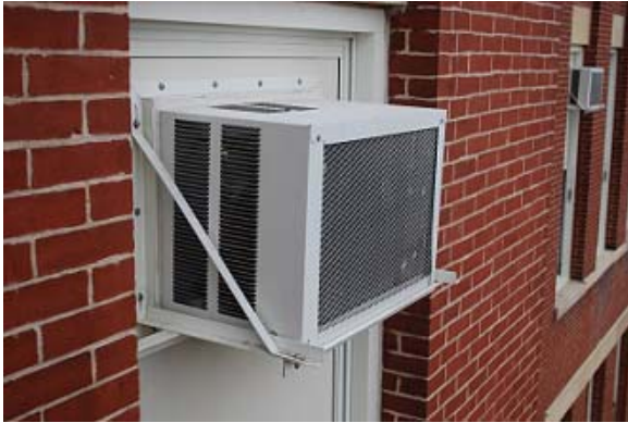
Typical Window A/C Installation
