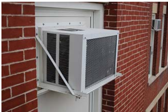
Typical Window A/C Installation
