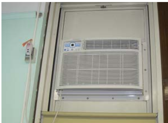
Typical Window A/C Installation
