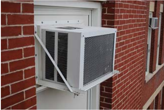
Typical Window A/C Installation
