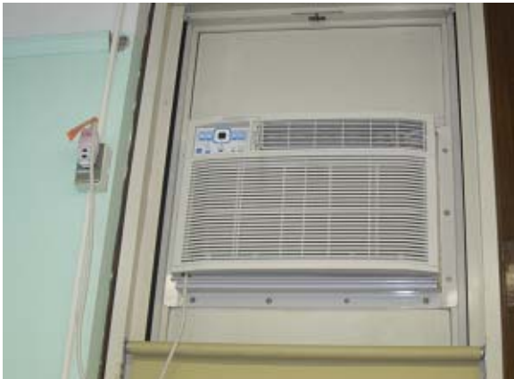
Typical Window A/C Installation
