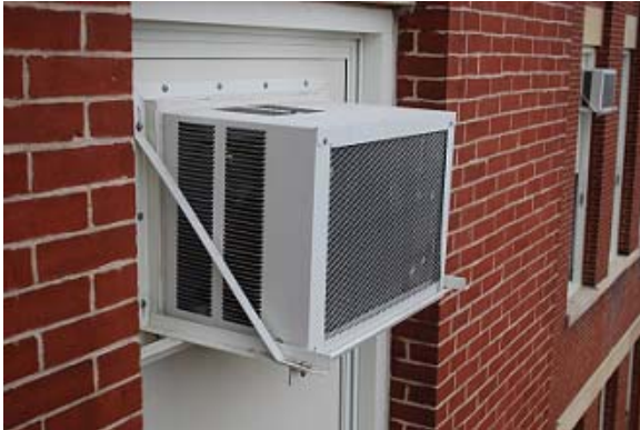
Typical Window A/C Installation
