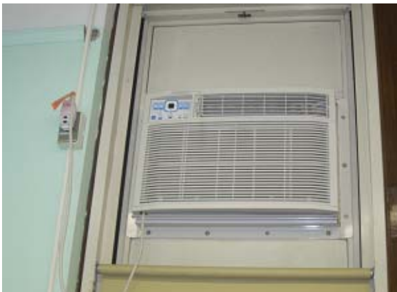
Typical Window A/C Installation
