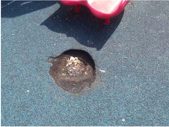
Current Surface Condition
