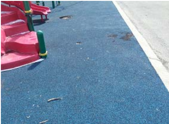
Current Surface Condition
