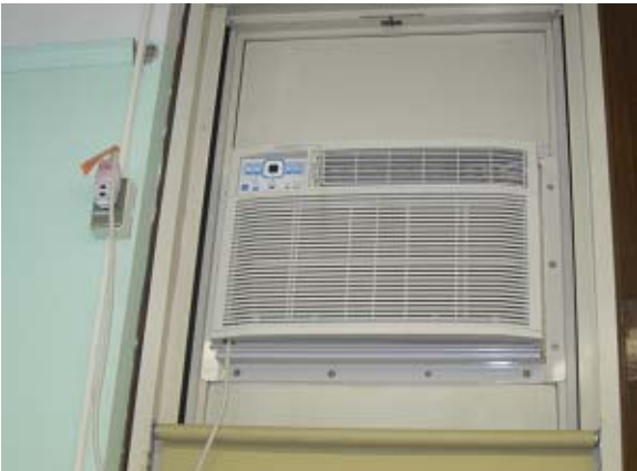
Typical Window A/C Installation
