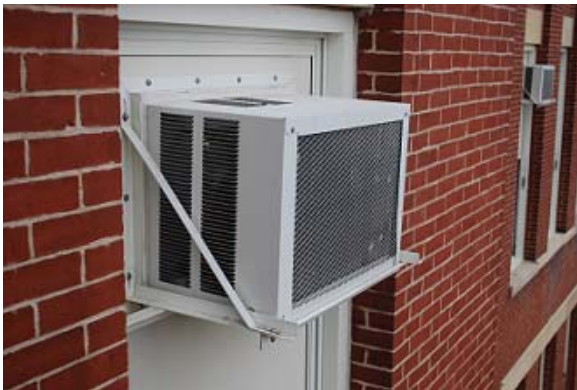
Typical Window A/C Installation
