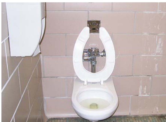
Provide ADA accessible toilet.
