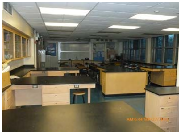
Provide ADA accessible sink.
