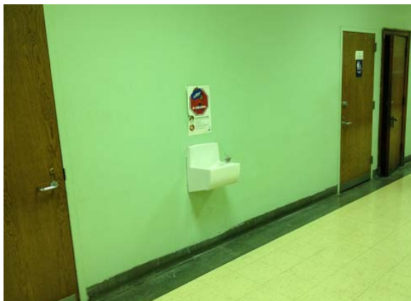
Replace non ADA compliant fountains.
