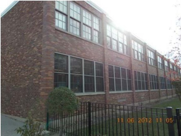
New window AC units
