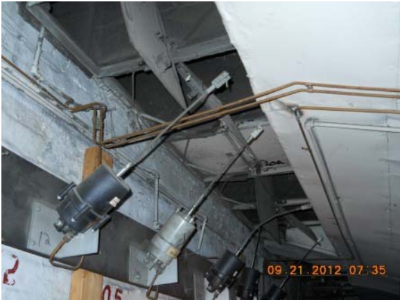
Repair mechanical systems
