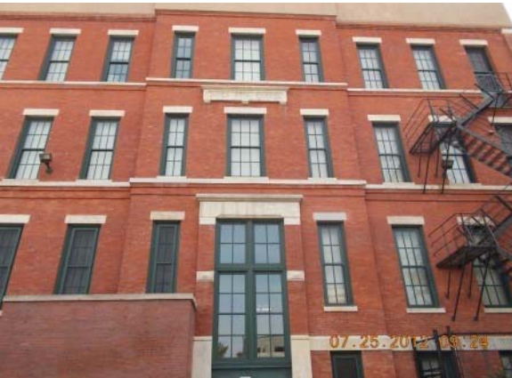
New window AC units
