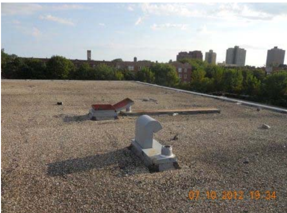
Replace annex roof.
