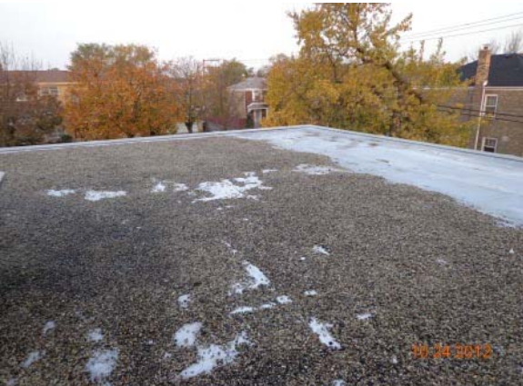
Missing ballast on roof.
