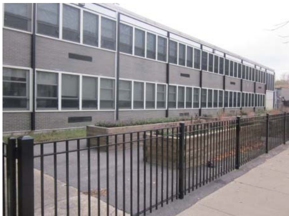
New window AC units
