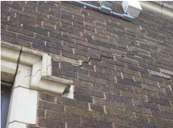
Targeted masonry repairs.
