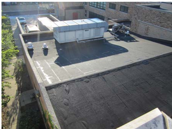
Patch bubbles in roof material
